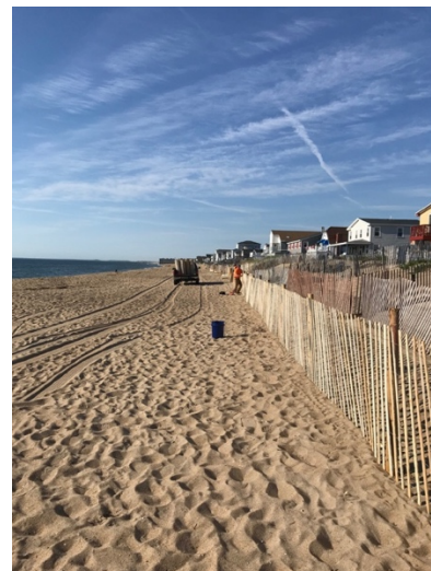
Contractors Installing Snow Fence on Salisbury Beach
